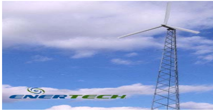
Figure 14. The 40 KW wind turbine. From [30]
